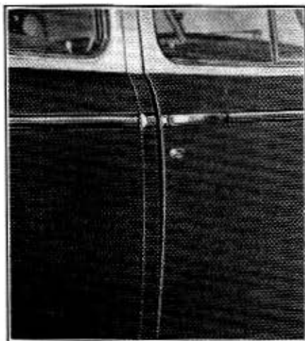
Fig. 1-95. A "bowed" door condition. Door fits at top and bottom, but stands away at the belt section.
